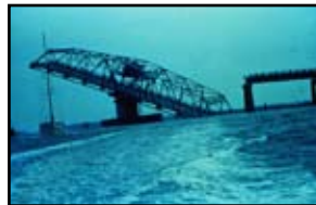
The Ben Sawyer Bridge to Isle of Palms, S.C., after Hurricane Hugo.
